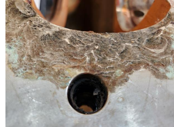
Close up of corroded area on the mating face
