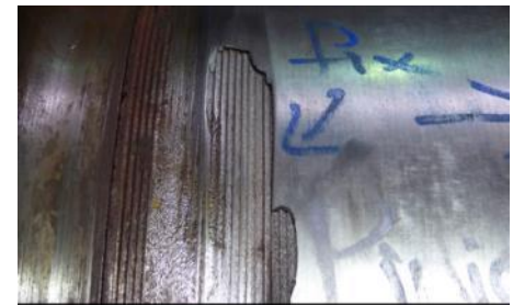
Failed repair work by others
