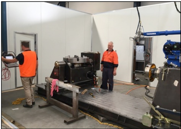
Pre Delivery Commissioning – Reviewing controls within enclosure prefabricated with safety interlocks.
